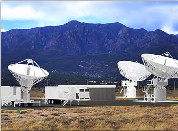
Figure 1: MET Terminal Antennas and Electronics Buildings
